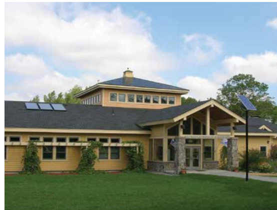
The George Robert White Environmental Conservation Center (GRWECC) is a LEED Platinum certified building. It consumes 30% less energy than a conventional building, uses fewer natural resources, and creates a safer, healthier space for occupants.
